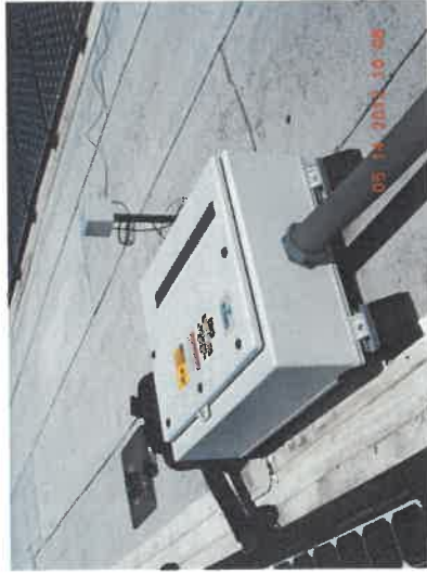
Figure 4-34 Measurement of Electric and Magnetic Fields near a Combiner Box on the Roof of the San Bernardino Solar Facility - The combiner box combines the DC outputs of multiple solar panels together and feeds current through the large conduit down to a ground mounted inverter.
