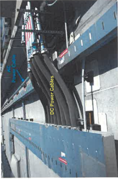
Figure 2-7 AC and DC Power Cables at Northeastern Rooftop Collection Area
