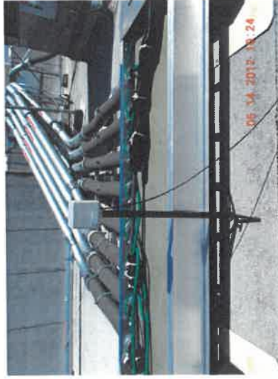
Figure 4-34 Measurement of Electric and Magnetic Fields near a Combiner Box on the Roof of the San Bernardino Solar Facility - The combiner box combines the DC outputs of multiple solar panels together and feeds current through the large conduit down to a ground mounted inverter.
