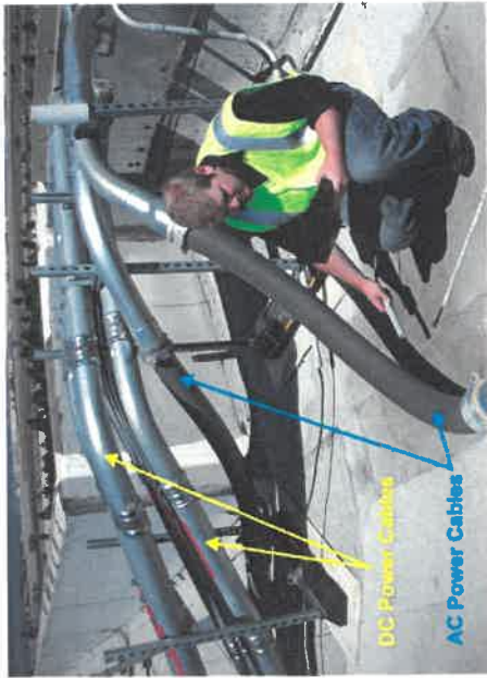
Figure 2-7 AC and DC Power Cables at Northeastern Rooftop Collection Area
