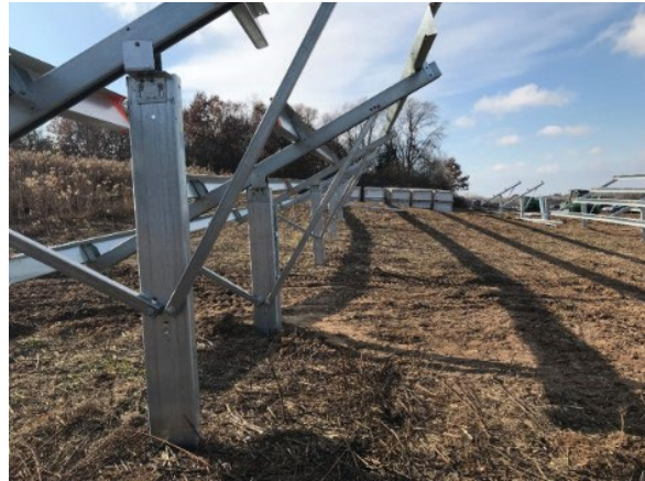
Example array construction showing pile being driven (left) and racking before module install (right)
