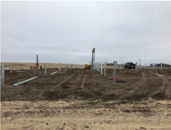
Example array construction showing pile being driven (left) and racking before module install (right)
